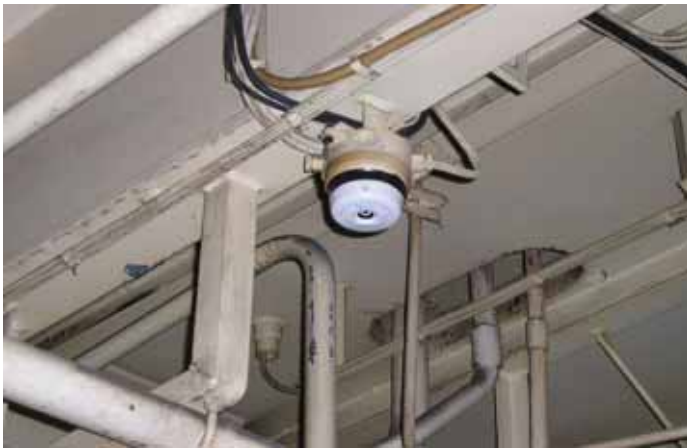
Identification and location of various fire sensors in the E/R between frames, pipes and cables
